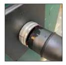
Apply silicone grease to the cone and insert into the extension flue piece.
