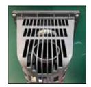
Instal flue terminal with the 4 screws supplied.
